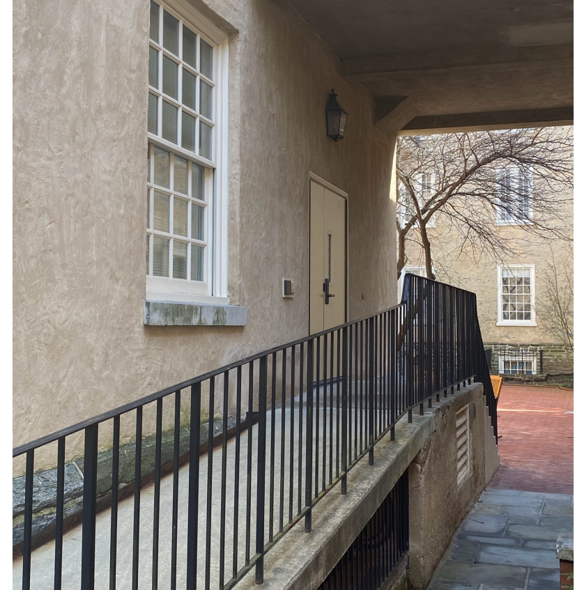
Only accessible entrance to Founders Hall
