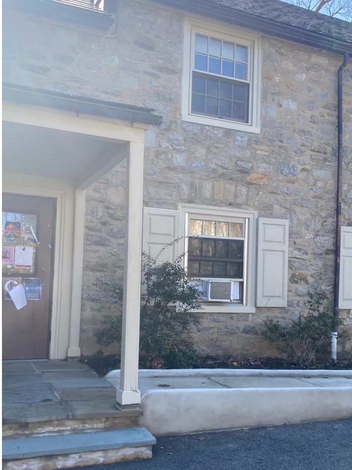
Entrance to Leeds Hall
